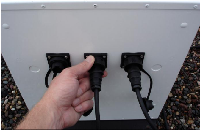
Figure 48: Connect Solar Cells to Battery Enclosure Box
