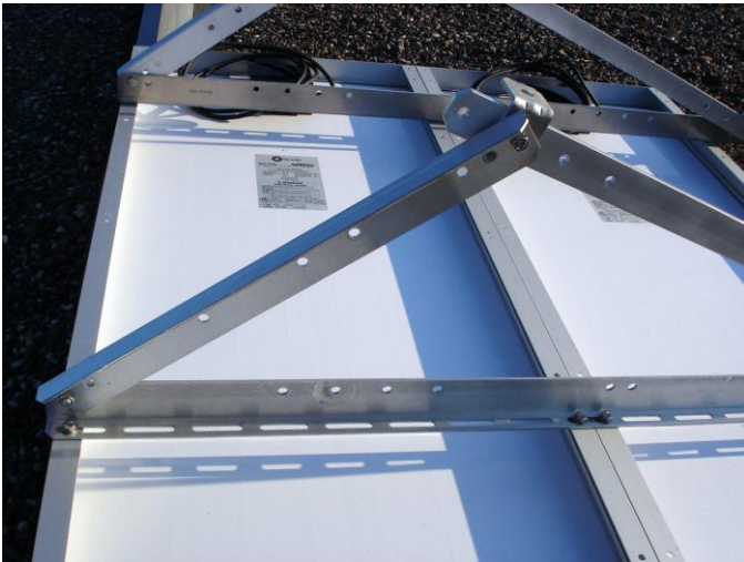
Figure 46: Assemble the Solar Cells on the Mounting Frame
