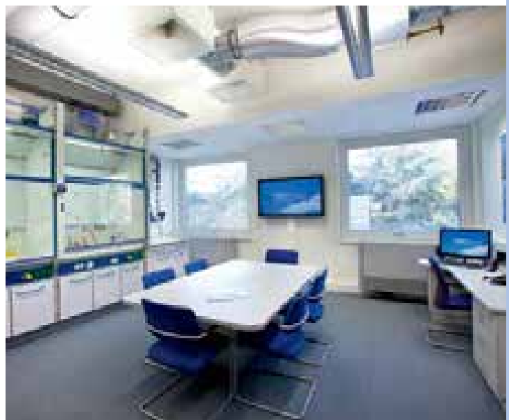
System demonstration in the TROX laboratory, Neukirchen-Vluyn, Germany
